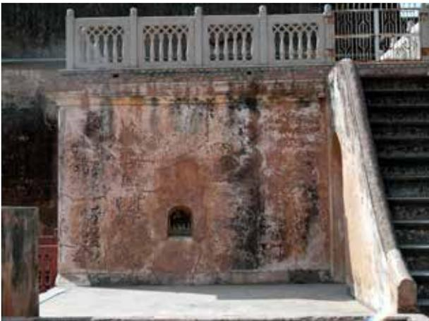
**This part of the foundry contains the melting chamber and has walls of around 1 metre thick. The small arched access hole is closed off with an iron plate operated by a lever set in the roof. The railing on top is a modern addition**
