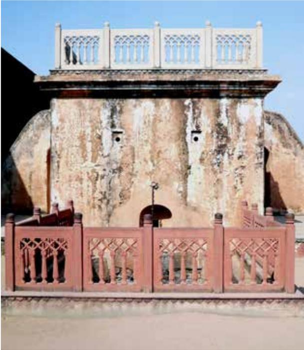
The front of the furnace with the 'tapping' arch and the casting pit behind the modern railing
