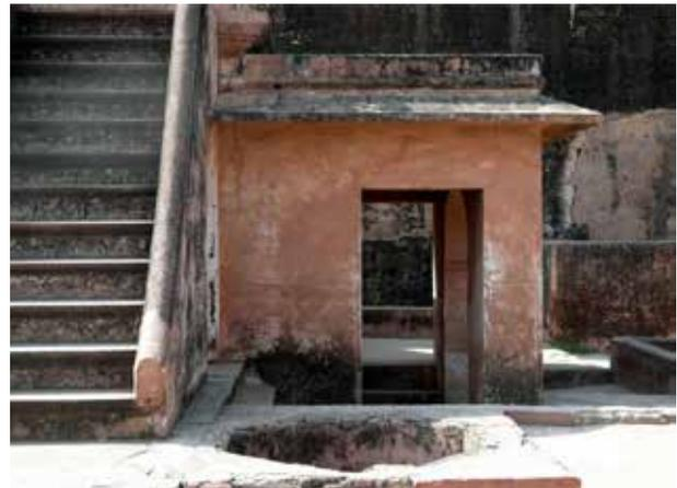
**The rear of the foundry - an open structure which surrounds the opening to the firebox**
