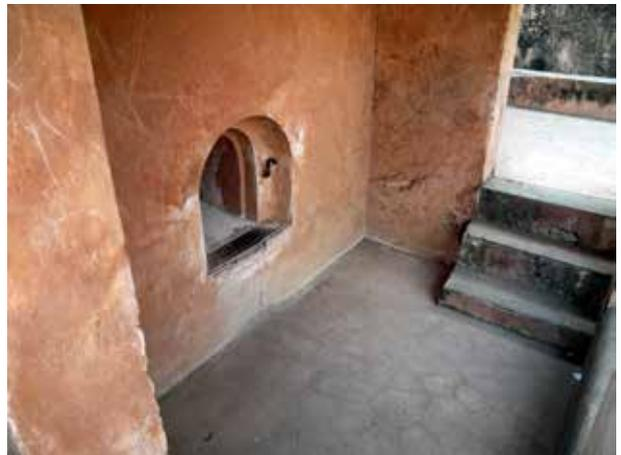
**The opening to the firebox at the rear of the foundry - the iron hooks would hold a locking bar to hold a door in position**
