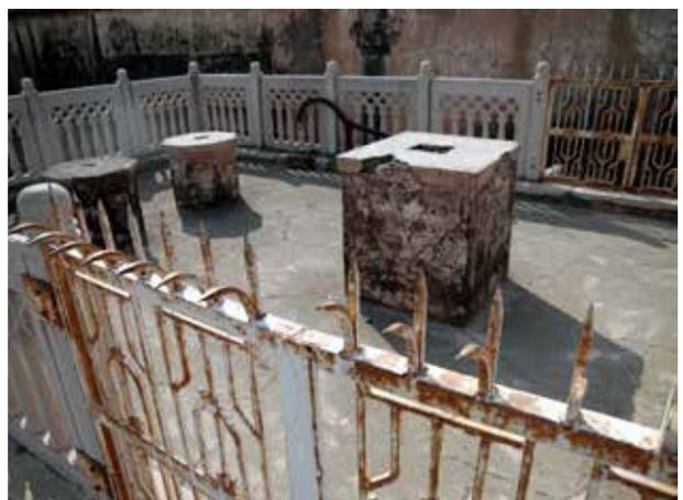
The chimneys - the two on the left are above the melting chamber, that at the rear is above the firebox
