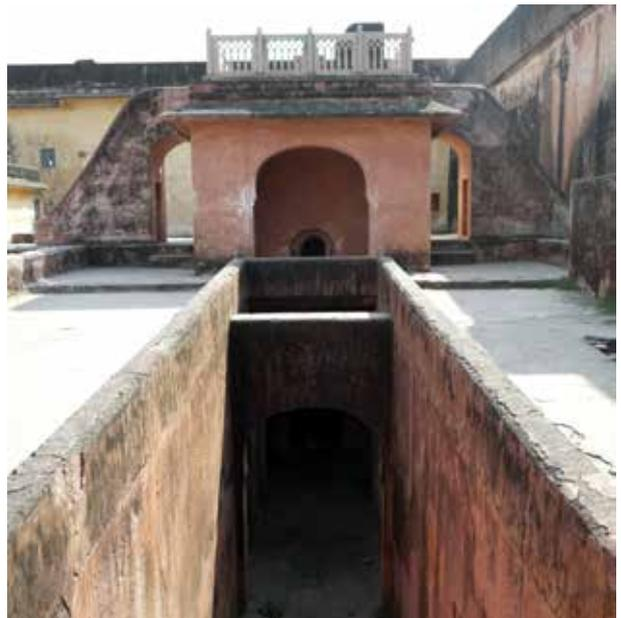
**The air passage under the foundry which provides an air draft for the fire**
