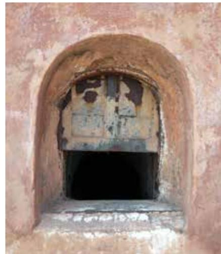
The charging hole in the side of the furnace. The metal door is operated by a lever set into the top of the furnace
