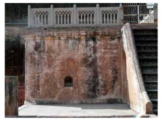
This part of the foudry contains the melting chamber and has walls of around 1 metre thick. The small arched access hole is closed off with an iron plate operated by a lever set in the roof. The railing on top is a modern addition
