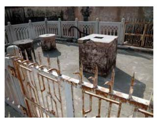
The chimneys - the two on the left are above the melting chamber, that at the rear is above the firebox
