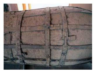
Detail of the iron reinforcing straps showing the way they were tightened around the moould using wedges to draw the ends together
