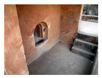
The opening to the firebox at the rear of the foundry - the iron hooks would hold a locking bar to hold a door in position
