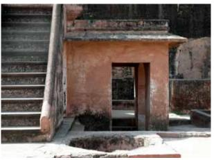
The rear of the foundry - an open structure which surrounds the opening to the firebox
