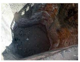
Looking down into the casting pit. Although it is now roughly octagonal, it appears that it was originally circular
