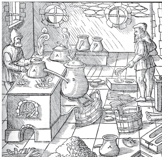
Refining sulphur - an illustration from Agricola's De Re Metallica .
