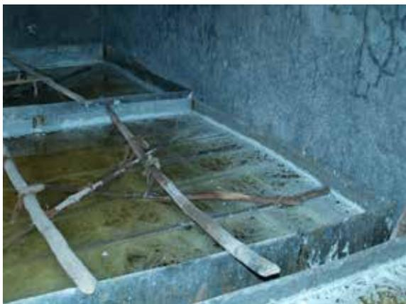
**Figure 25. A precipitation tank with a lattice of bamboo on the surface of the liquid**
