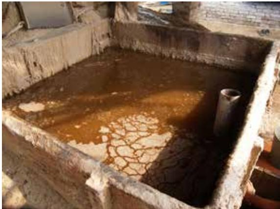
**Figure 23. The settling tank**
