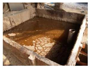
Figure 23. The settling tank
