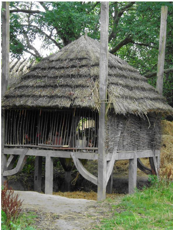
**Figure 1. The nitre bed with the chicken house built over it**
